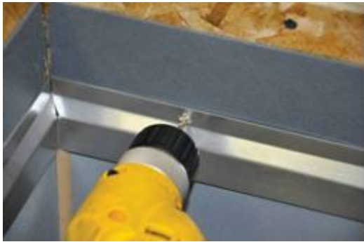
Pre-drill using 1/8" drill bit
