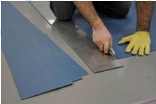
Turning 5' x 8' sheets into 6" x 8' strips
