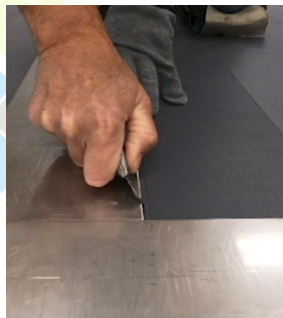
Using a knife and straight edge for repairs
