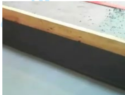
Finished flash cove
