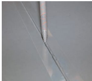
Rapid Weld dispensed into groove
