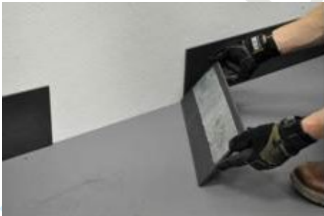
Using web reinforced tape
