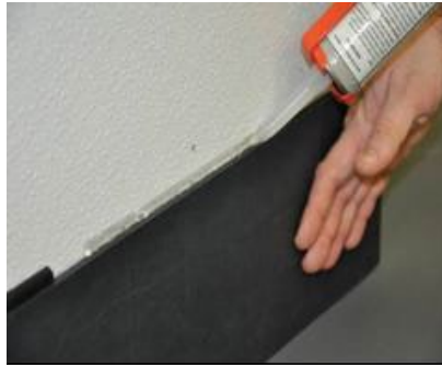
E6100 applied to top of base metal
