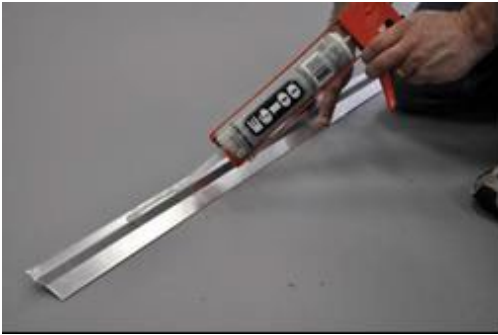
Seal back of cove cap with E6100 before securing to wall
